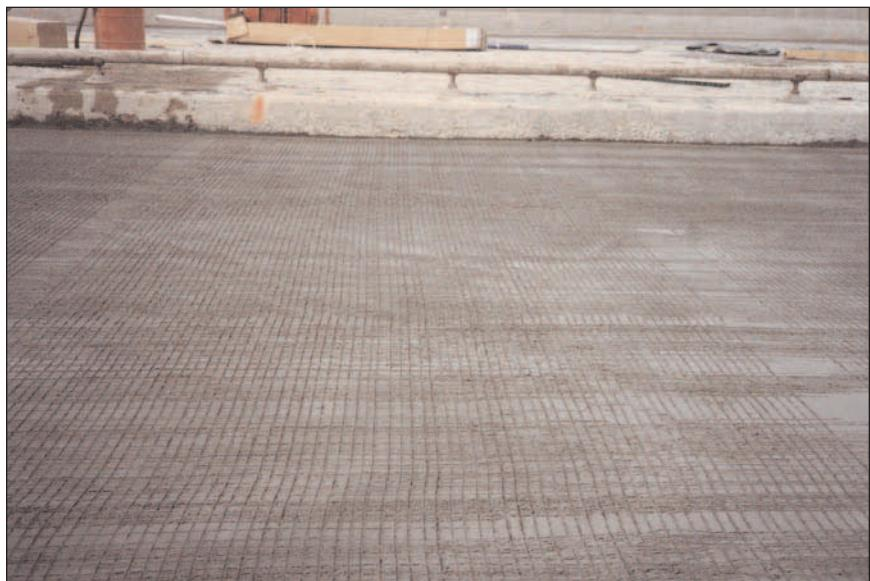
**FIGURE 8.10C.** Surface of a properly tined deck.
