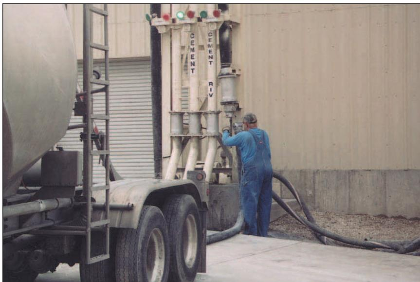
**FIGURE 7.5B.** Connecting rubber hose from tanker to rubber fill hose of silo.
