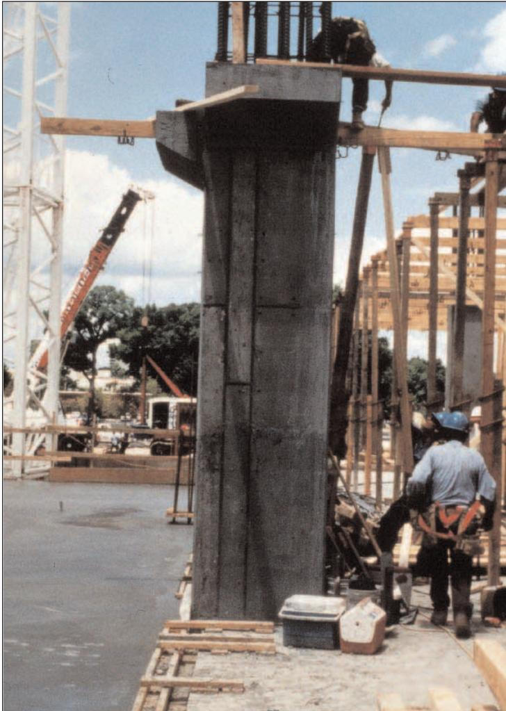
**FIGURE 6.5.** High-strength columns project. Mixture proportions for a concrete that could be used on this project are developed in Example 3.
