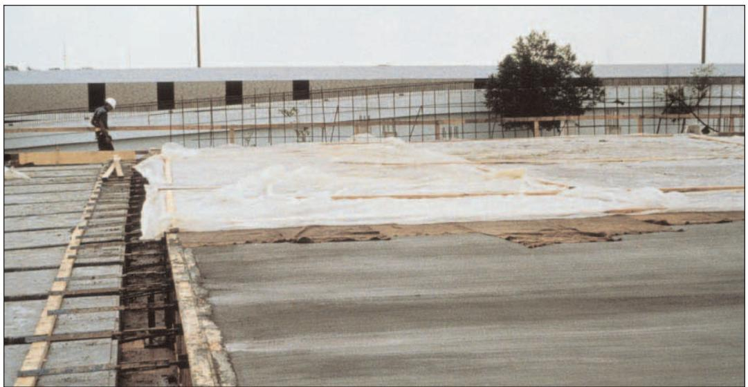
**FIGURE 8.18B.** Burlap and plastic sheeting used for final curing. For most applications of silica-fume concrete, wet curing will provide better in-place concrete quality than the use of curing compound alone.
