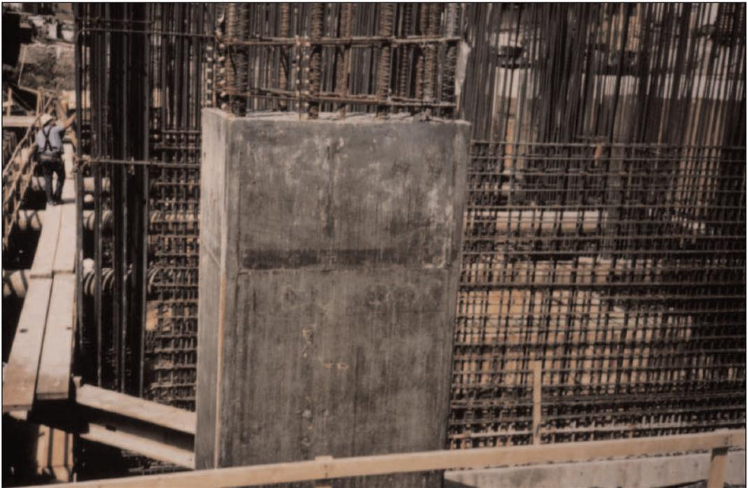
**FIGURE 3.7.** High-strength silica-fume concrete column in a high-rise structure.
