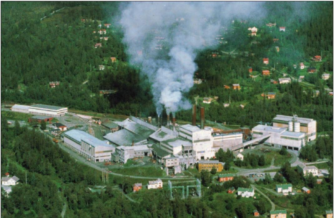
**FIGURE 1.2.** Smelter before installation of equipment to collect silica fume. The “smoke” is silica fume being released to the atmosphere. Today, in the U.S., no silica fume is released — it is all captured and used.
