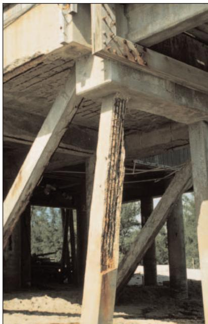
**FIGURE 3.13.** Corrosion damage to a marine structure.
