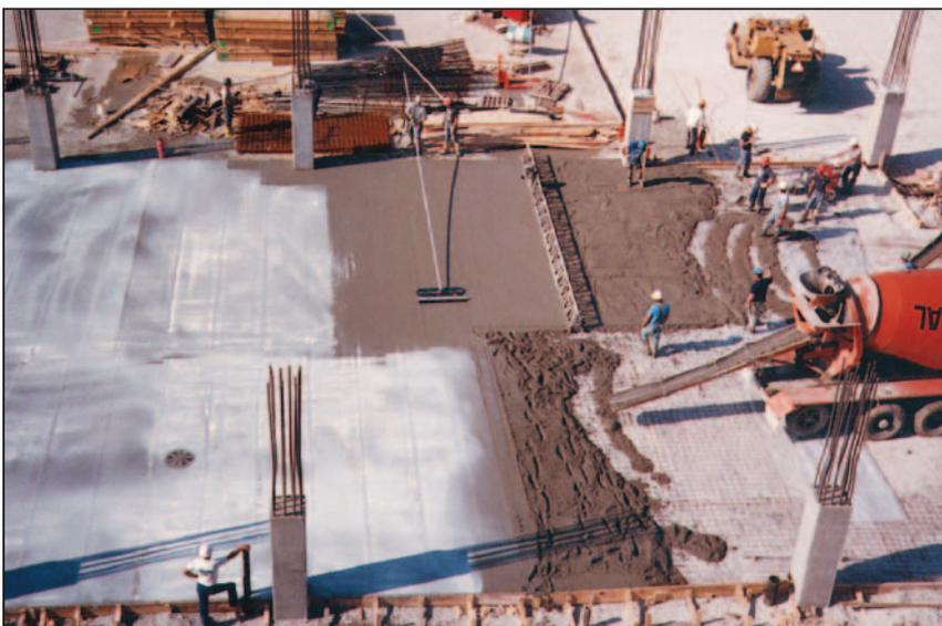
**FIGURE 8.12.** One-pass finishing. Concrete is being placed, screeded, floated, textured, and cured without any waiting between operations.
