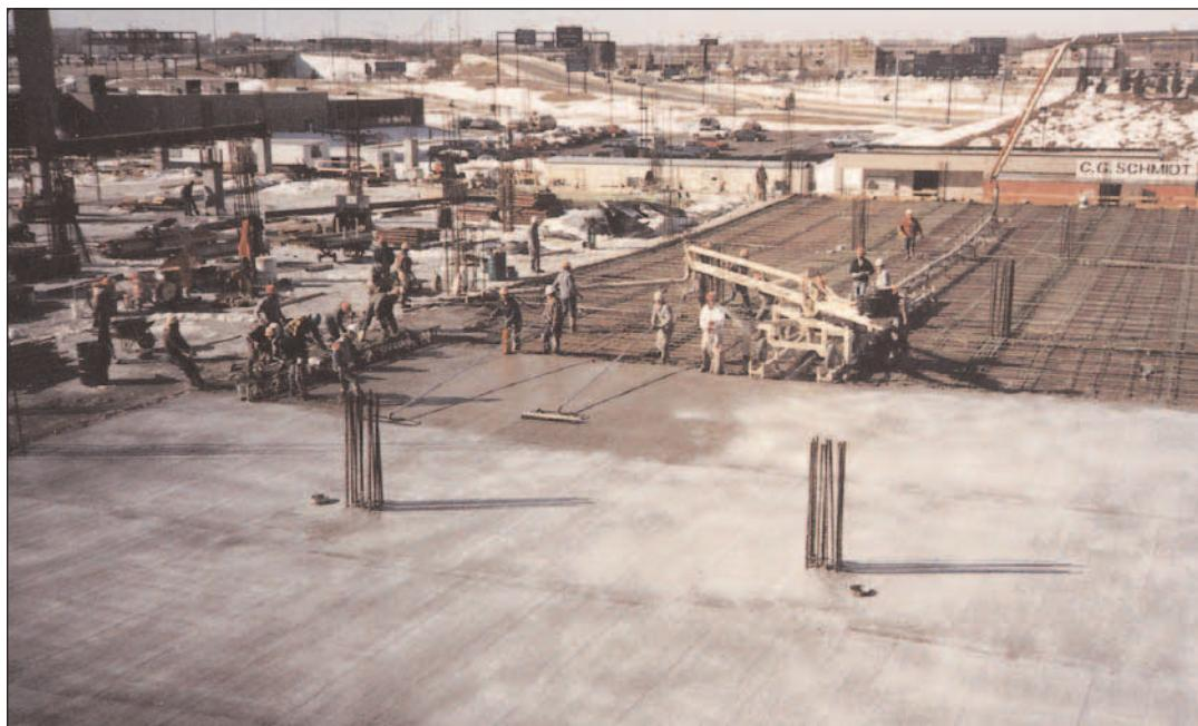
**FIGURE 3.4.** “One-pass finishing” of silica-fume concrete in a parking structure. Placing, finishing, texturing, and curing are done as a continuous process.
