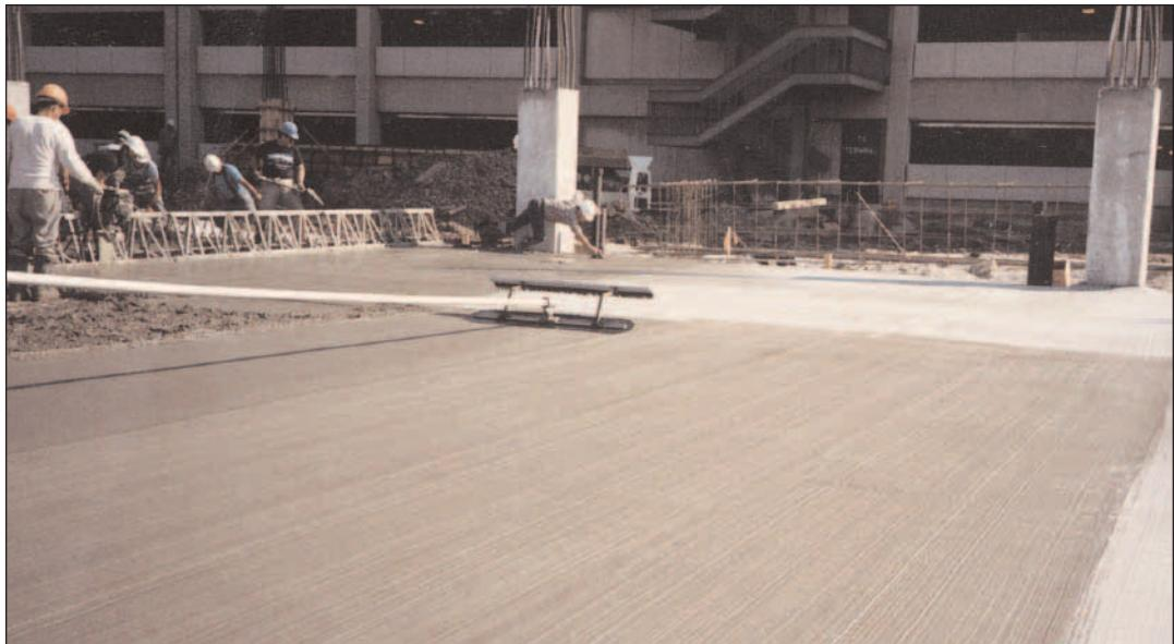
**FIGURE 8.17B.** This photo shows a finishing tool that is a combination of a float and a broom. In one direction, it serves as a float. In the other direction, it serves as a broom.
