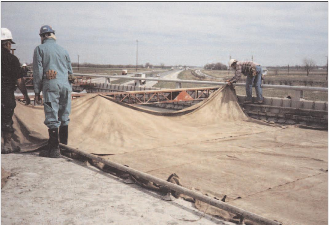
**FIGURE 8.11C.** Curing silica-fume concrete bridge deck. Applying wet burlap.
