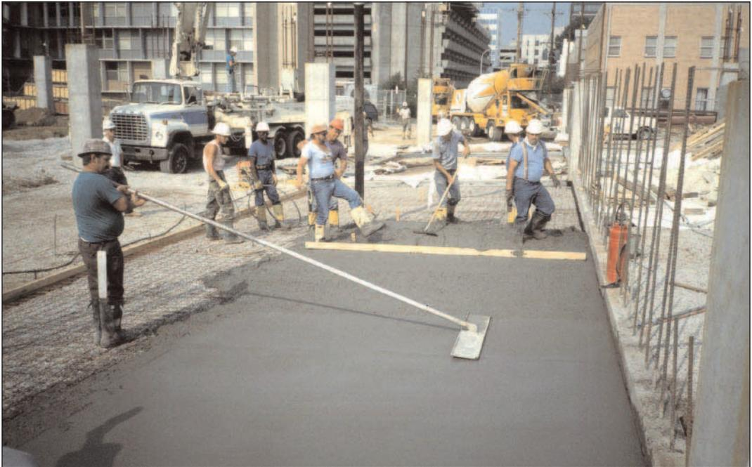
**FIGURE 8.14.** Conducting a trial placement using the one-step finishing procedure. Note that the trial is a slab on ground on the actual structure. Note that placing the wire mesh on the bottom of the slab is not recommended practice.
