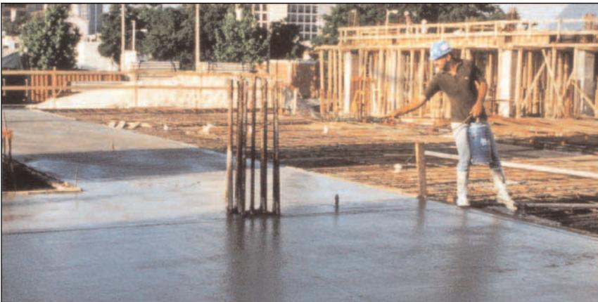
**FIGURE 8.5.** Applying evaporation retarder to silica-fume concrete to prevent loss of moisture before curing begins.
