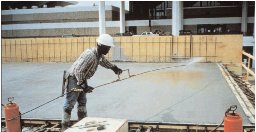
**FIGURE 8.18A.** Curing compound is being applied to silica-fume concrete in a parking structure shortly after brooming. In many cases, the use of curing compound is the preliminary curing method; it is intended to protect the concrete until it gains enough strength to allow placing wet curing materials on the deck without marring the surface. On this particular project, wet burlap and plastic sheeting were used for the final curing.
