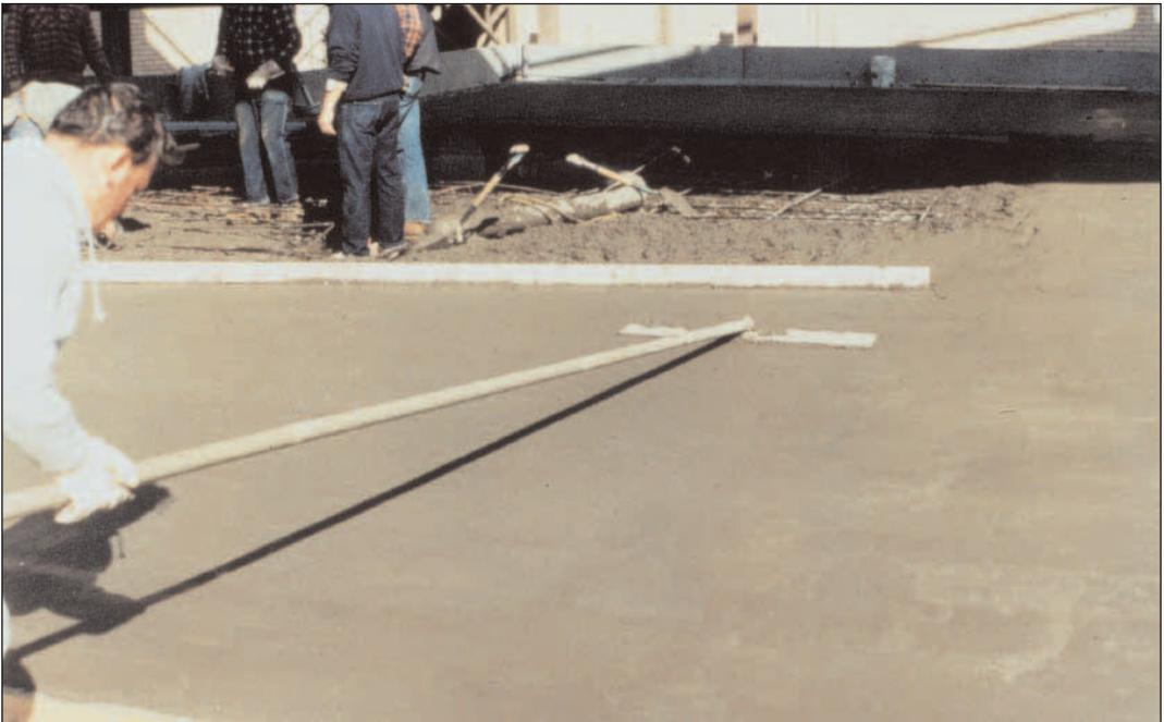
**FIGURE 8.17A.** Depending upon the nature of the surface finish selected, it may be necessary to perform one additional pass with a float before the surface texture is applied.
