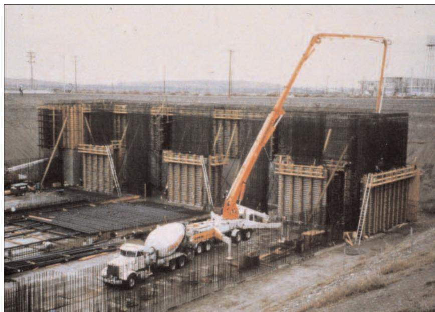
**FIGURE 3.16.** Concrete containing portland cement, fly ash, and silica fume being placed. The fly ash was used to control heat of hydration while the silica fume provided early strength required for stripping forms. For more information on this project, see the article by Holland (1998).
