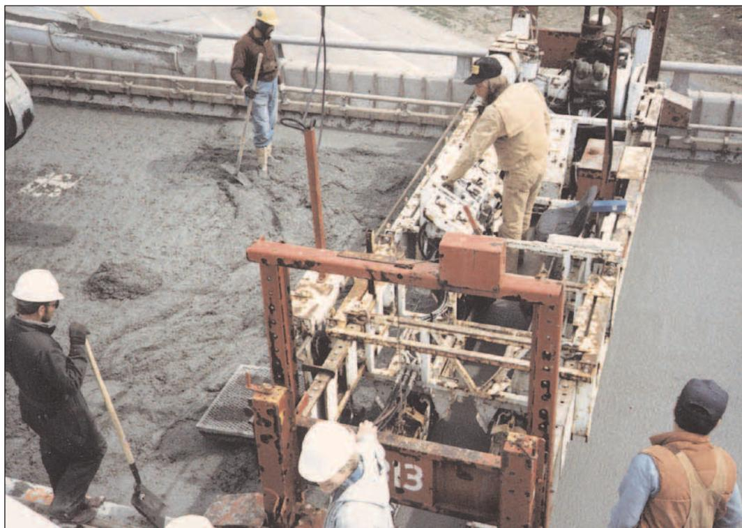
**FIGURE 8.9.** Bridge deck machine being used to place silica-fume concrete overlay.
