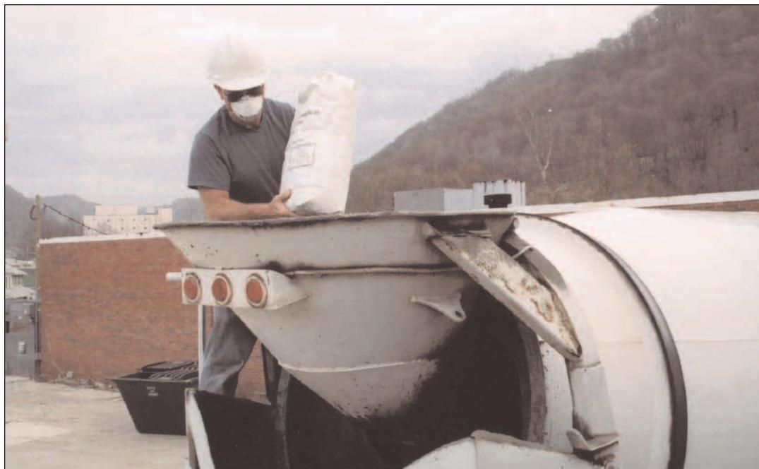
**FIGURE 7.6.** Adding repulpable bags of densified silica fume directly to truck mixer. See Section 7.3 for precautions regarding unopened bags. Note the use of a dust mask and safety glasses. See Chapter 9 for personal safety recommendations.
